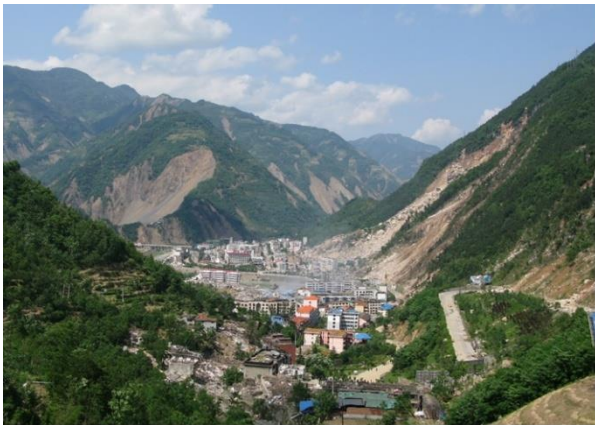
Fig. 4 Widespread slope failures in 2008 Wenchuan Earthquake
